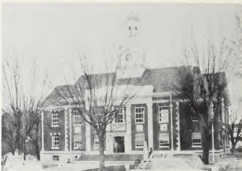
Cannon County Courthouse, built in 1935-1936.
